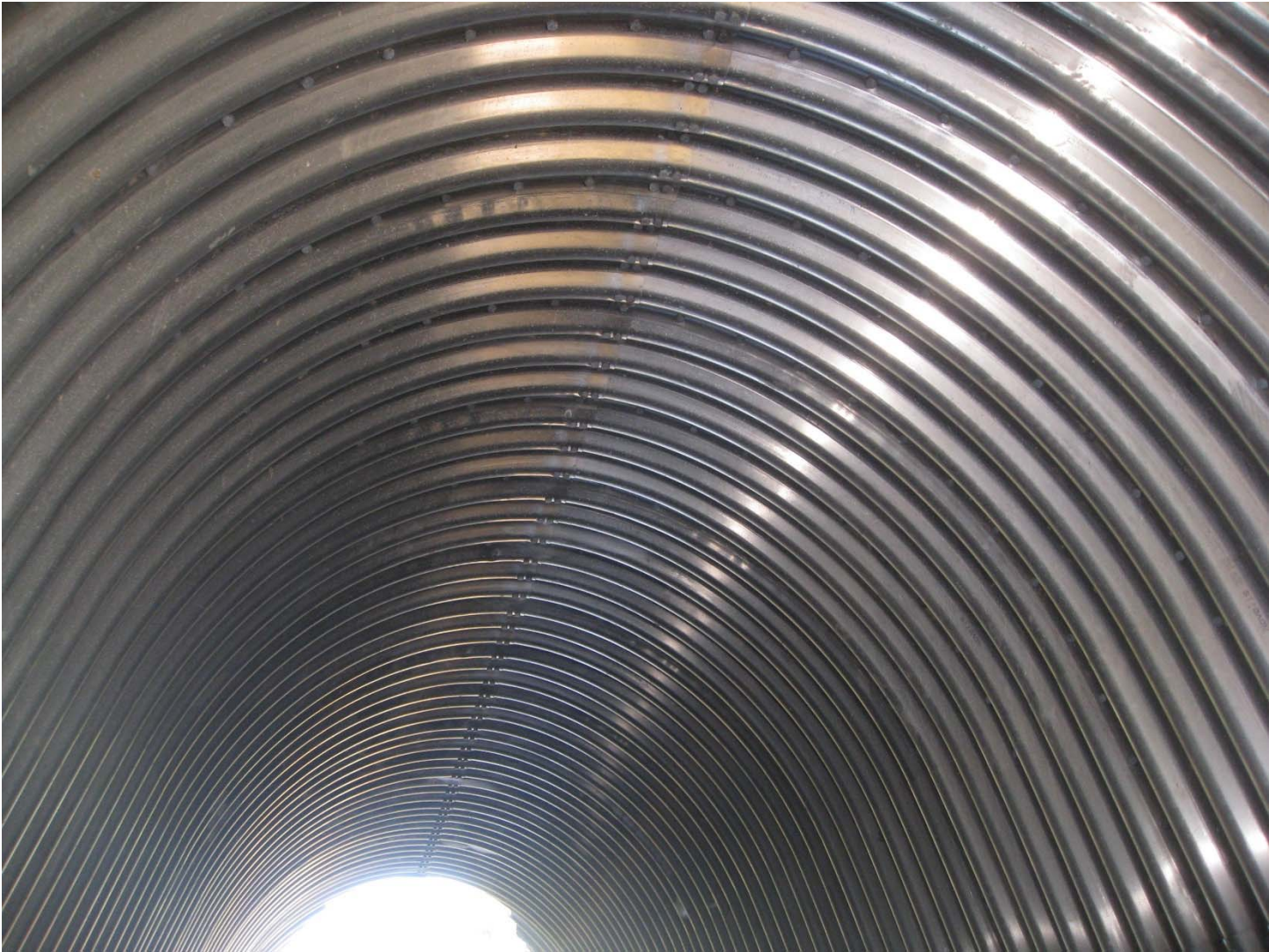
Photo 3 Interior ceiling of the culvert looking West
