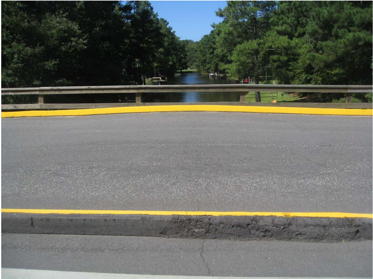
Photo 2 Centerline of culvert looking West
