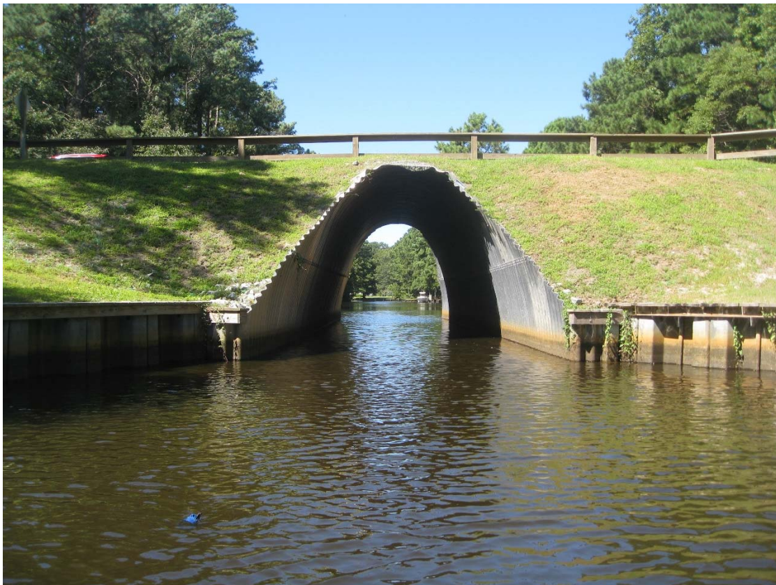
Photo 1 Juniper/Trinitie Trail Culvert looking West
