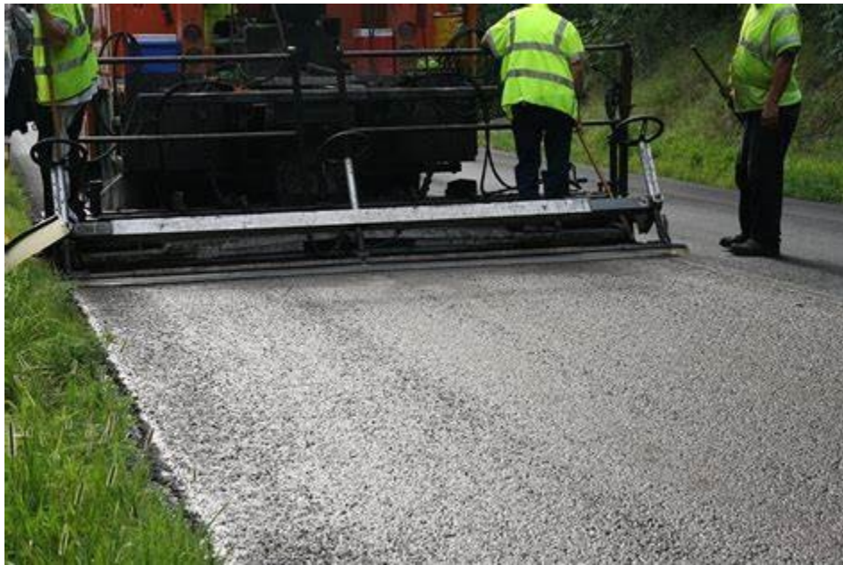
Figure 18: Typical Microsurfacing Paving Crew
