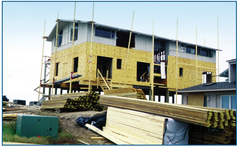
Figure 4 Vertical addition to a home damaged by Hurricane Fran. Pre-existing 1-story home became the second story of a home elevated to meet new foundation and floor elevation requirements.
