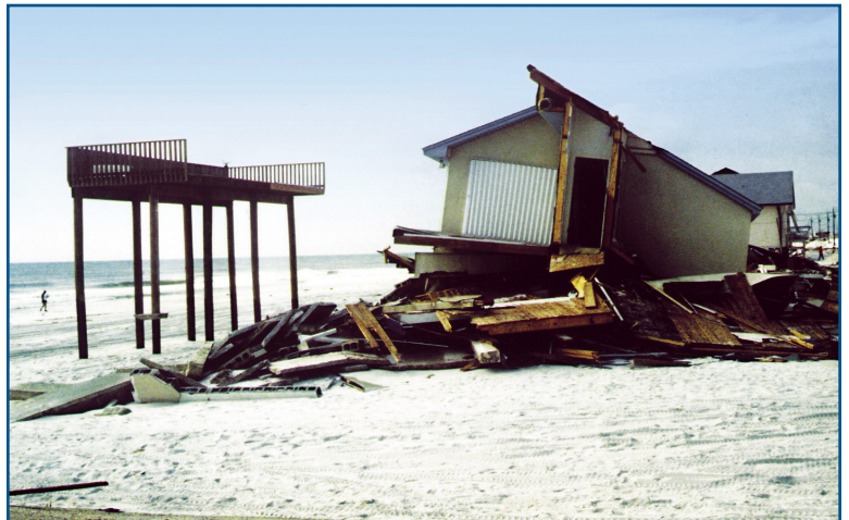
Damage from Hurricane Opal in Florida. This deck was designed to meet State of Florida Coastal Construction Control Line (CCCL) requirements. The house predated the CCCL and was not.
