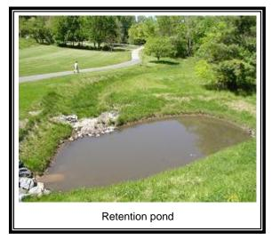
Flood control reservoirs are most commonly built for one of two purposes. Large reservoirs are constructed to protect property from existing flood problems. Smaller reservoirs, or detention basins, are built to protect property from the stormwater runoff impacts of new development.
