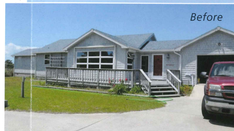
Older home in Hatteras village elevated to mitigate flood risks
