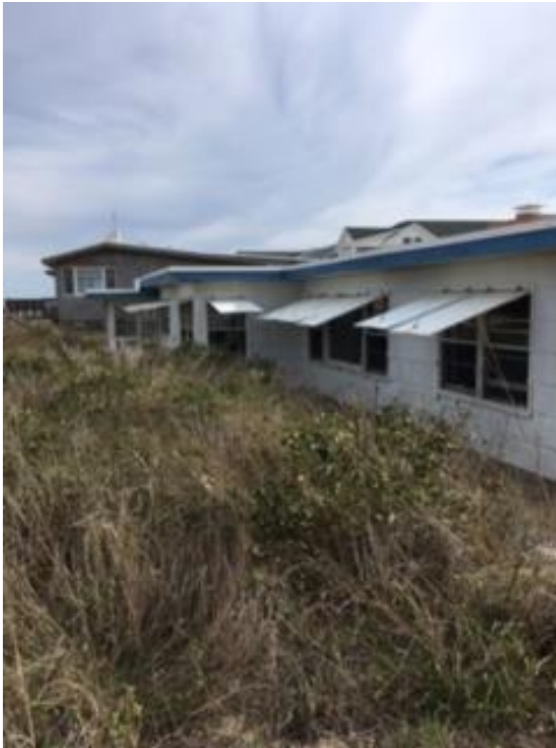
Mackey Cottage, East Facade
