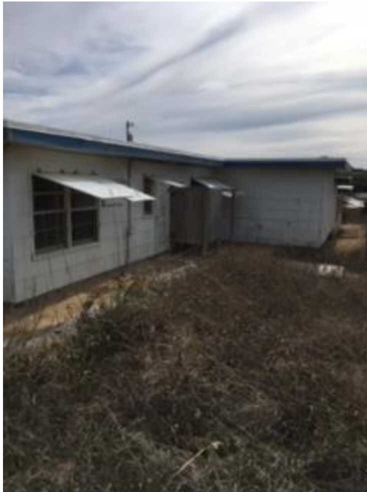
Mackey Cottage, North Facade
