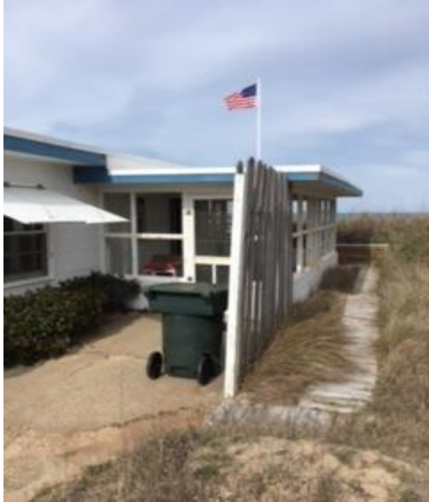
Mackey Cottage, South Facade
