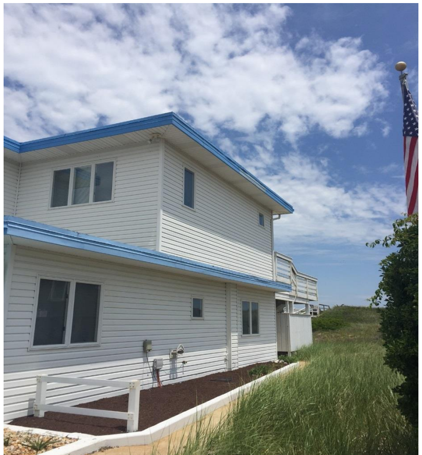
Figure 3: South side of 142 Ocean Blvd
