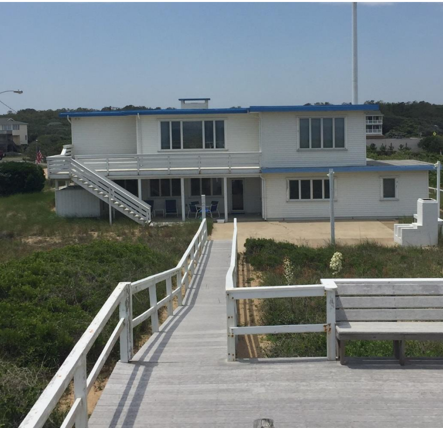
Figure 5: The east side of 142 Ocean Blvd that displays the second story addition and back deck that was added in 1980.
