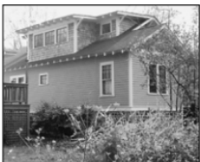
This upper floor attic addition echoes the design details of the original bungalow while respecting and retaining the original roof ridge line and eaves.
