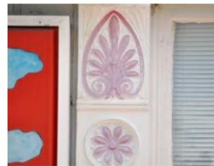
Detailing on Metal Pier
