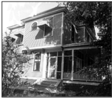
A sensitively designed second-story addition to the front side elevation of this residence projects slightly beyond the screened porch over which it sits.
