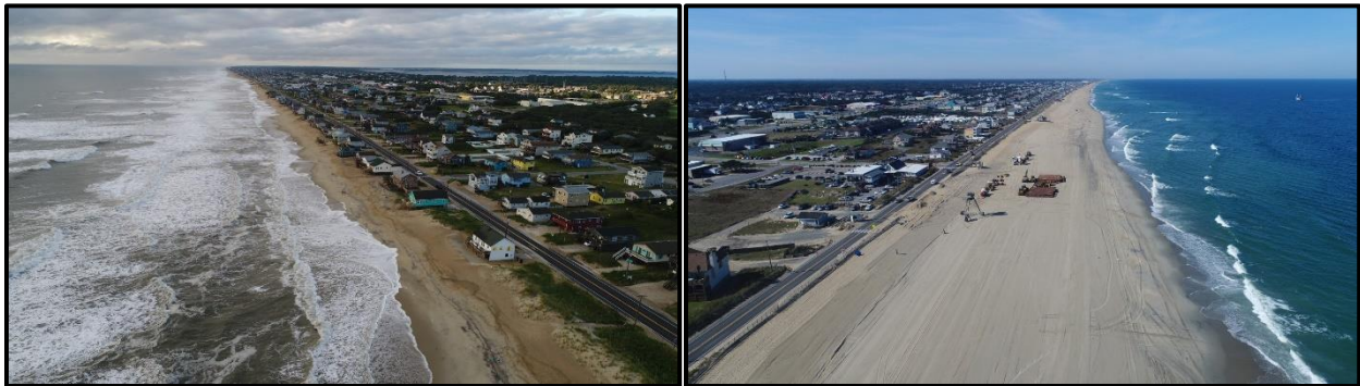
Figure 8. View of the beach nourishment project within the Town of Kitty Hawk, Pre-Construction (left), Post-Construction (right).
