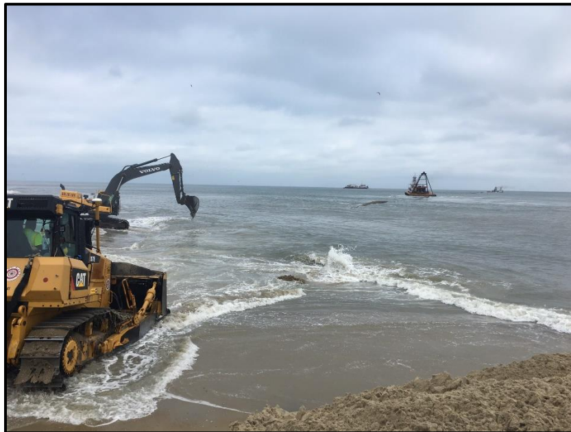
Figure 13. Subline at Lillian Street being uncovered on October 11, 2017.
