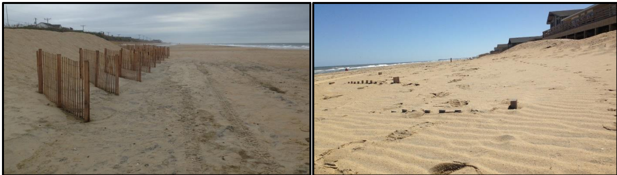
Figure 12. View of the accumulation of sand near the installed sand fencing at White Road in Kitty Hawk prior to (left) and after (right) the storms that affected the Dare County project in September 2017.
