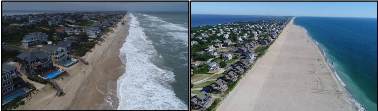
Figure 6. View of the beach nourishment project within the Town of Duck, looking north - Pre-Construction (left), Post-Construction (right).
